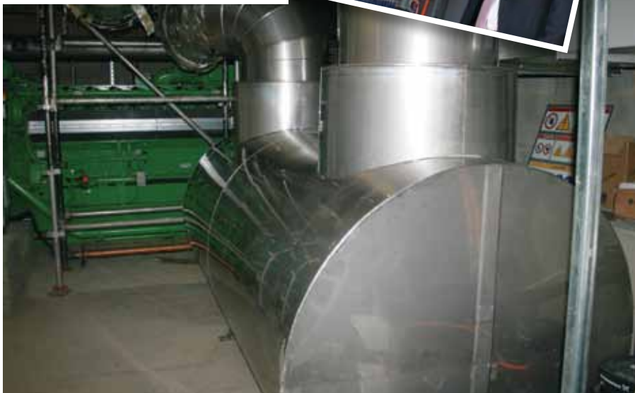
Waste heat is ducted away for reuse; Tom Russell (L) and RSL chief Richard Eddington.
