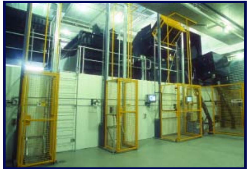
Wastech Engineering was forced to create a unique lift system at the main waste dock to raise transit bins to the compactor.
